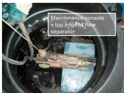
Inspection of flushing results with pan and tilt camera, camera on the maintenance console in the start shaft of a SediPipe L system
