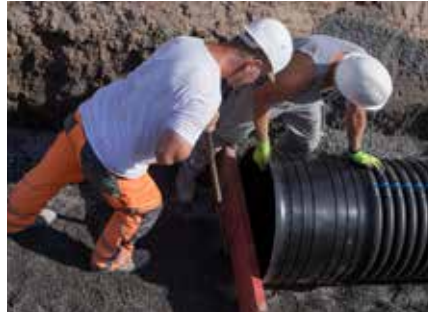
4. Installing the sedimentation pipe
