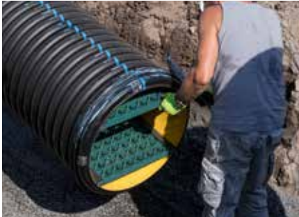
3. Applying lubricant onto the sealing ring
