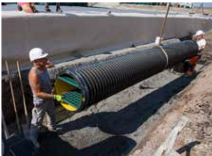
2. Moving the sedimentation pipe to the installation position
