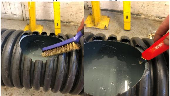
The seal was then inserted into the 170mm hole and lubricant applied to the internal sealing faces. The 160mm pipe leading edges were chamfered to aid insertion into the seal and the seal was inserted to the required 95mm design depth. The final 10mm was only achievable by using a block of wood on the end of the 160mm plastic pipe with a hammer.
