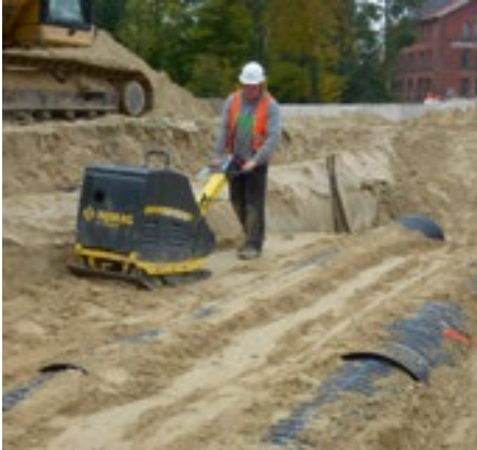
Compacting of lateral backfilling
