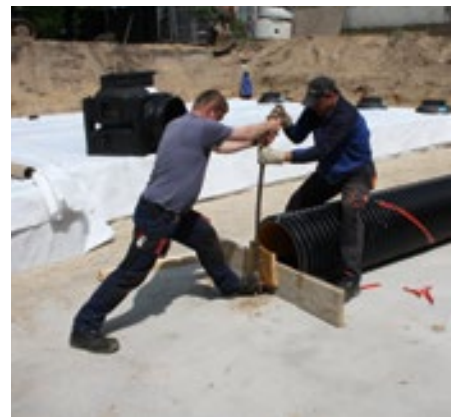
Installation of sedimentation pipe
